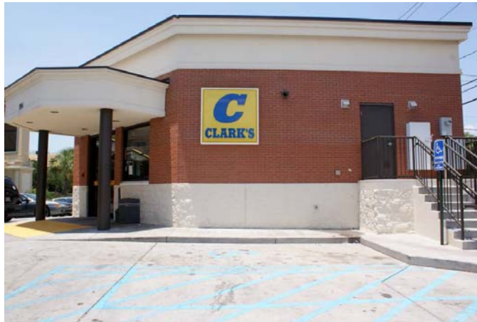
Fig. 3.5. PHOTO: Dry floodproofed structure in East Biloxi.
