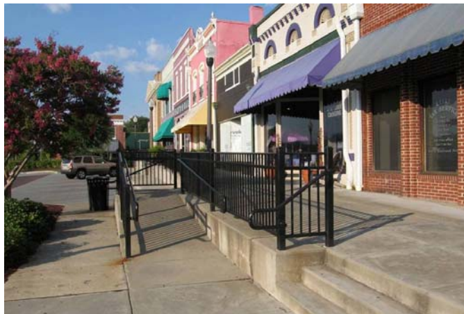
Fig. 3.7. PHOTO: Shared, elevated walkway with ramp and stair access.
