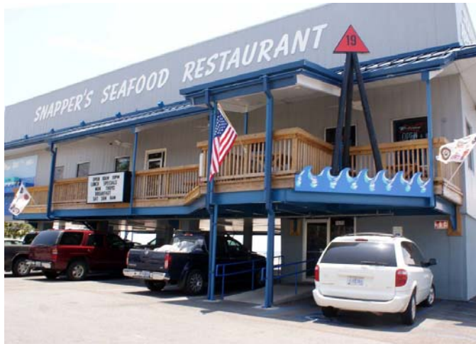
Fig. 3.3. PHOTO: Visual access problems associated with an elevated structure.
